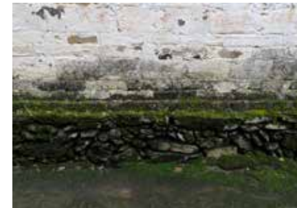
BLUESTONE SLAB In the past, bluestone slabs were excavated and transported from the surrounding mountains. These slabs are used for foundations, paving, and bridges. They have been preserved for a long time. The ancient stone bridge in Xixi Village was built 300 years ago.
