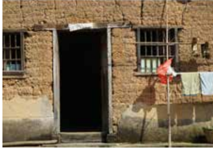
RAMMED EARTH Rammed earth is a traditional local building material. Rammed earth buildings have the characteristics of local materials, simple construction, warm in winter and cool in summer, and low cost. But there are very few rammed earth buildings in these four villages now.
