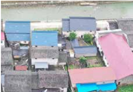
IMITATION GLAZED TILE & ALUMINUM TILE Most of the new houses built after the 1980s use these two types of tiles. It is worth mentioning that because of the price, the villagers did not use real glazed tiles, but imitated glazed tiles with clay inside and colored outside.
