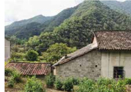
BLUE TILE Blue tile is the most common type of tile, which is made from clay. Blue tiles are divided into plate tiles and tube tiles. The old houses in these four villages all use plate tiles. In the past, Xihu Township had a factory for making blue tiles, and the villagers bought it there.
