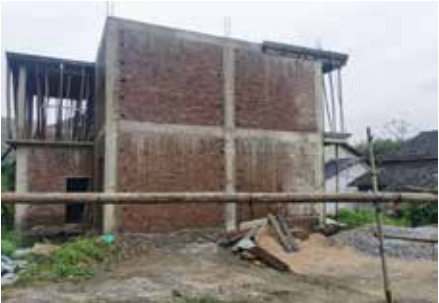
NEW BRICK Today's buildings mostly use brick-concrete structures. The bricks also use uniform red bricks, including solid bricks and hollow bricks. They are mainly purchased from the building materials market in Fuliang County.
