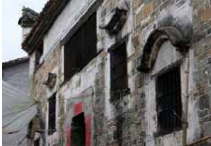
OLD RED OR BLUE BRICKS They were commonly used building materials in the past in the four villages, and the specifications and construction methods of these old bricks are different from those of new bricks now. And they mainly come from the old brick factories in Xihu Township.
