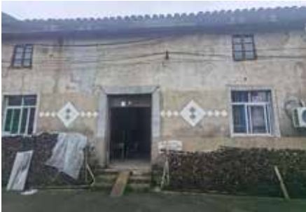
TERRAZZO & SWASH STONE Swash stone is a traditional construction technology, it can make the wall have a natural texture. It is made of crushed stone, mortar, glass slag and concrete. Mainly used for wall decoration. Terrazzo is similar to the water-brushed stone method, and will be polished at the end.
